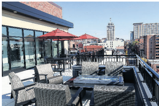
A top-floor terrace with fire pit is perfect for community or private gatherings.
